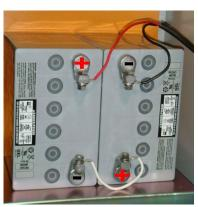
**STEP 8:** If batteries are installed on their side make sure to apply an insulator to the top of the battery terminal to prevent the battery terminals from shorting to the metal enclosure in case the battery shifts inside the enclosure during an earthquake.
