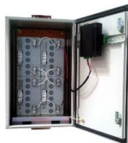
RPST with 200Ah of battery
