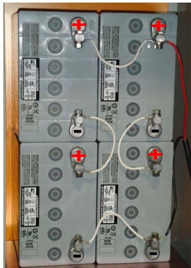
**STEP 8:** If batteries are installed on their side make sure to apply an insulator to the top of the battery terminal to prevent the battery terminals from shorting to the metal enclosure in case the battery shifts inside the enclosure during an earthquake.
