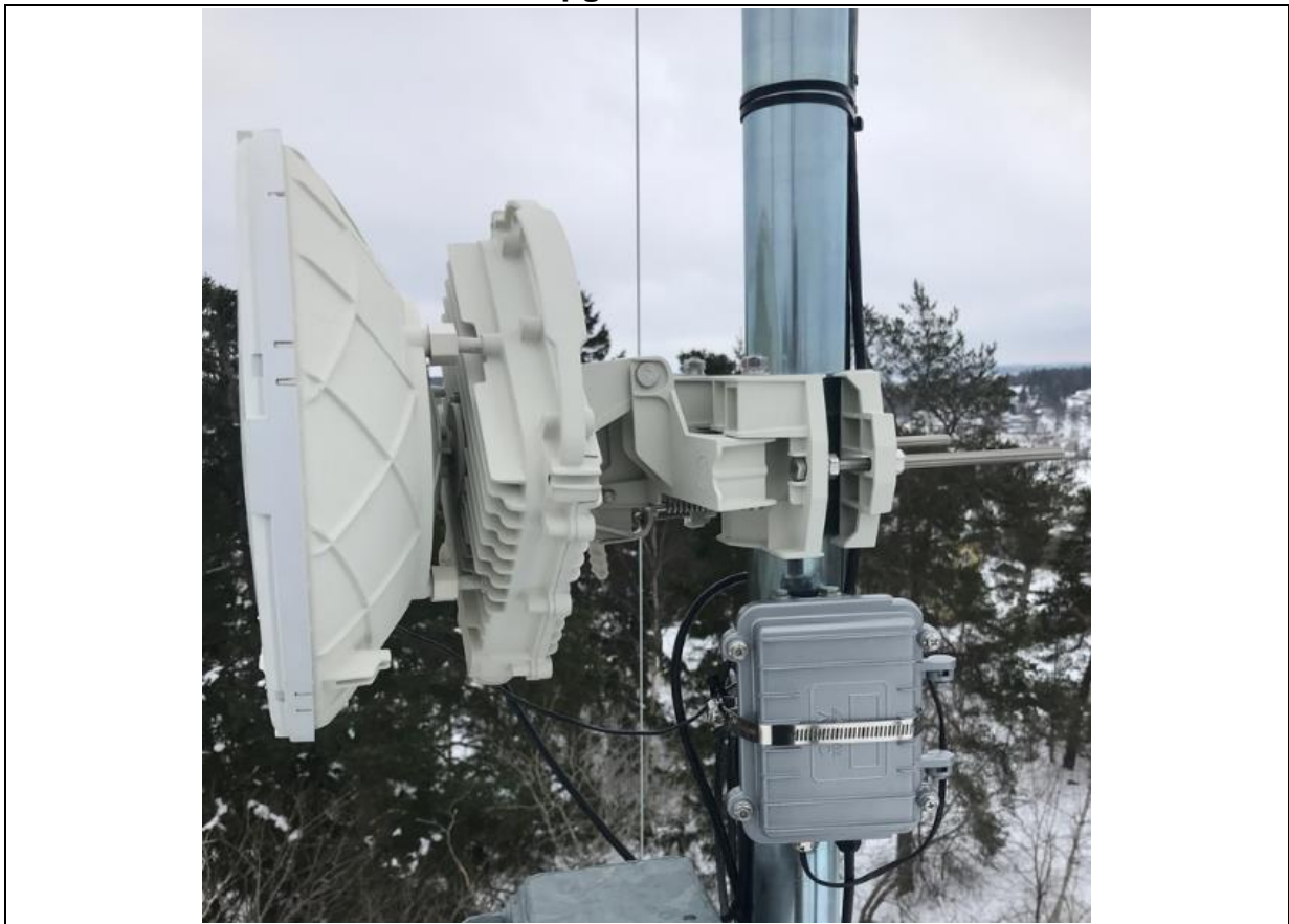
FIGURE 1a: EH-1200TX-ODU-1ft upgraded with EH-ANT-1ft-HR
