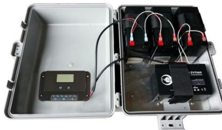
20A PWM Controller Inside
