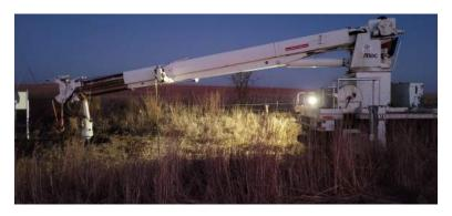
Step 2 & 3: Base Pole Section Set in Hole and Shimmed, Expanding Foamed Added
